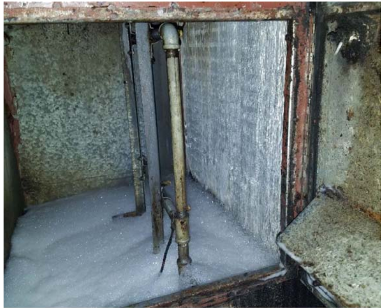
Figure 3: HRU washdown section showing clean coil.
